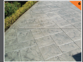
Finish Type: Stamped Surface Color Combination: Solid Color Stain Light Gray (275) Dark Gray (277) Product: Enhancer
